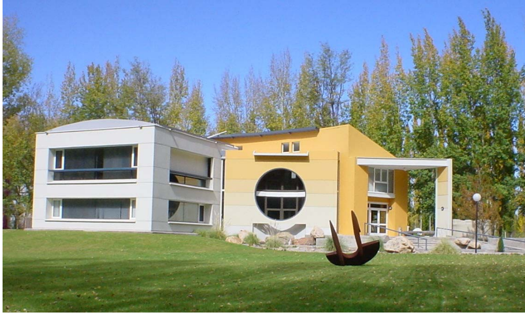
Office and CDAS building
